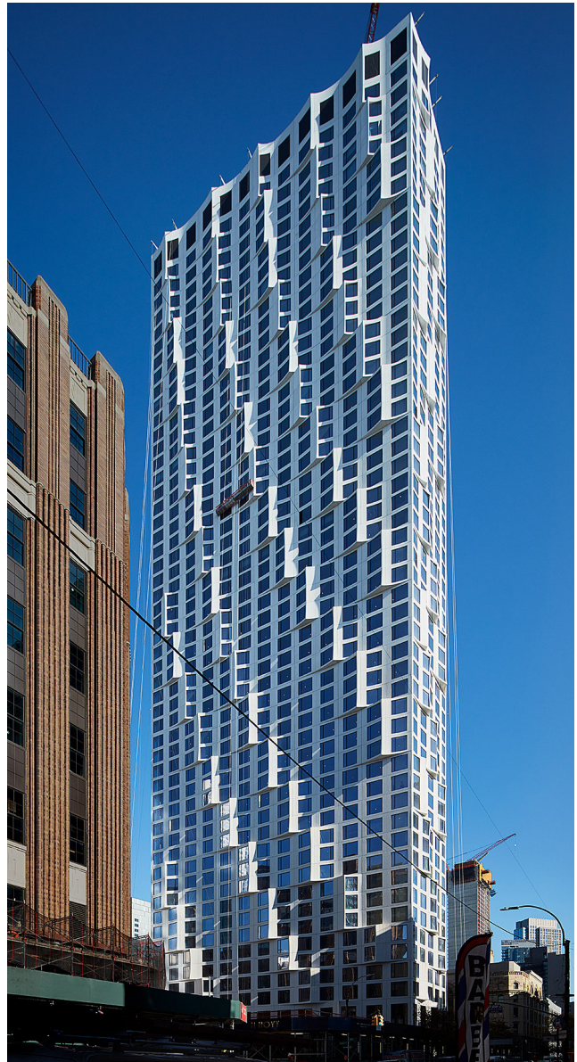
The system of precast concrete double-donuts used in the 11 Hoyt condominium tower facade was selected for its reliability and watertightness. The new Brooklyn, N.Y., structure contains 476 residential units. Copyright Tom Harris, courtesy of Studio Gang.
